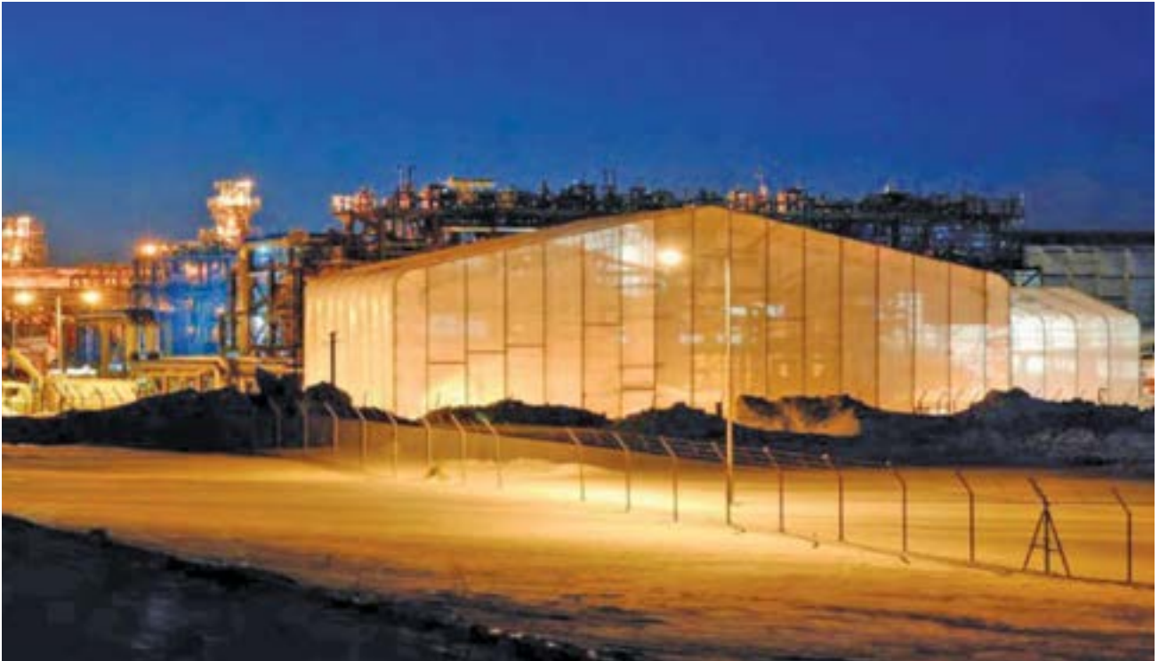
Processing compressor group covered via shelter type steel-structure supported textile
